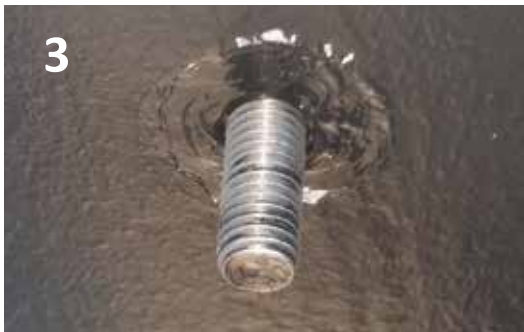
3 Use Sikaflex to seal the bolt M8
